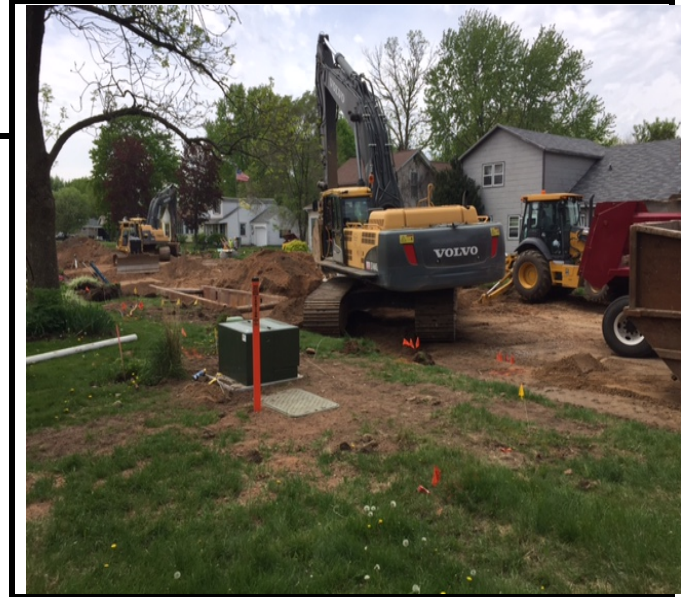
Two City crews installing underground utilities on 1 st St.
