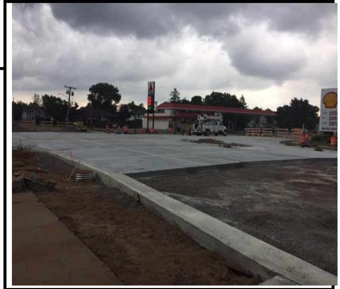
8 th St intersection at E. Grand nearing completion
