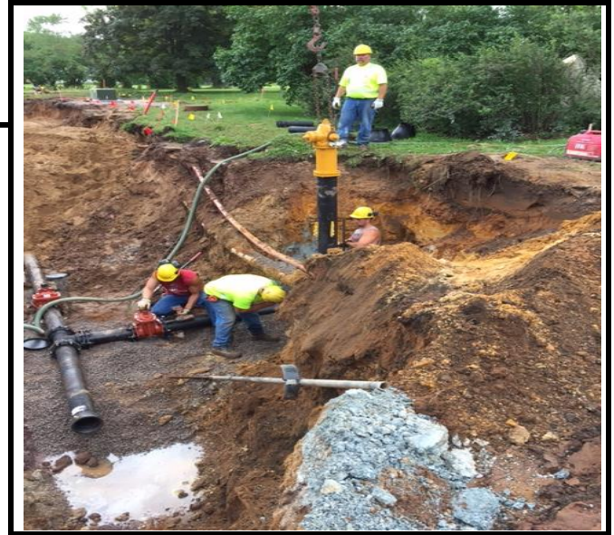
Watermain installation on 1 st St North
