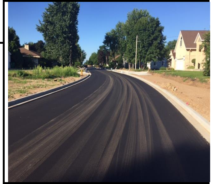
Binder layer applied to 800 feet of 1 st St North
