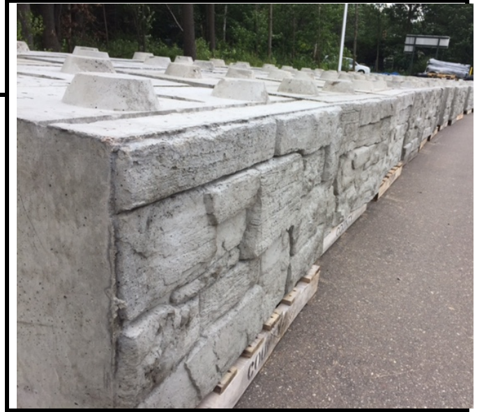
Retaining wall blocks arrive for North end of 1 st St.
