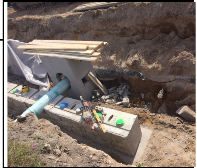
Retaining wall construction on 1 st St.
