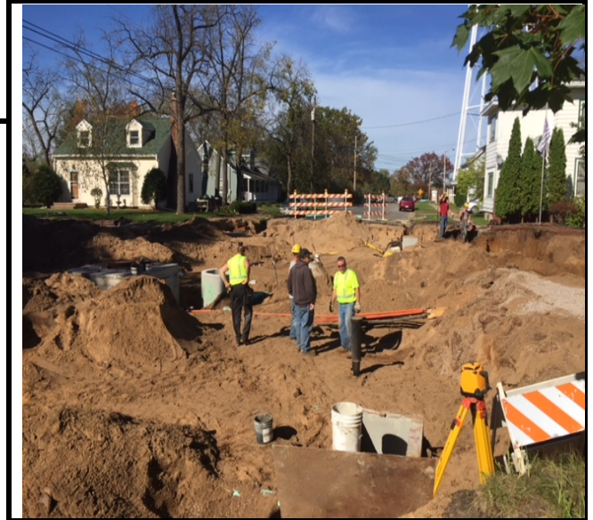
Workers survey the dig at 10 th & Washington St.
