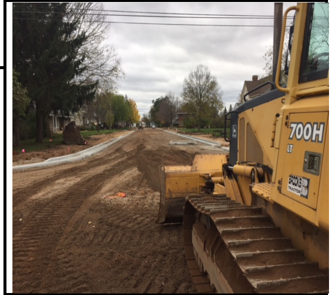
Excavation work wrapping up on Washington St.
