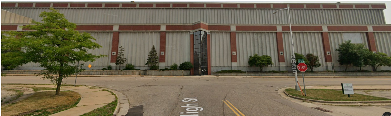
Figure 4 High Street Eastbound, Control: stop sign
