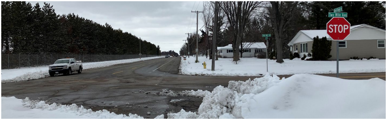
Figure 4 Airport Hanger Dr Northbound
