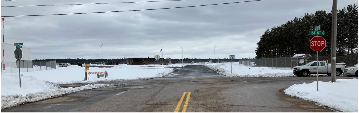
Figure 2 Two Mile Ave Westbound
