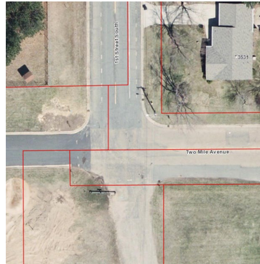
Figure 1 Intersection of Two Mile Ave and 1 st St S
