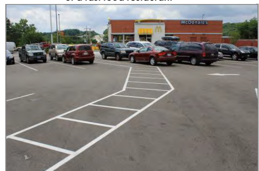
Exhibit 17-1. A pedestrian crosswalk in the parking lot of a fast food restaurant
