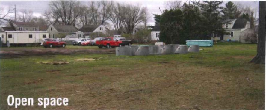
Park during utility work
