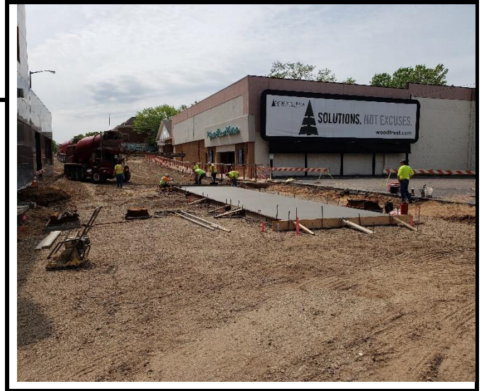
Pember Construction Co. completed first concrete pour on E Grand Ave.
