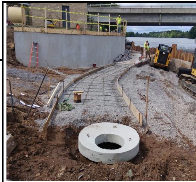
New retaining wall at Demitz Park
