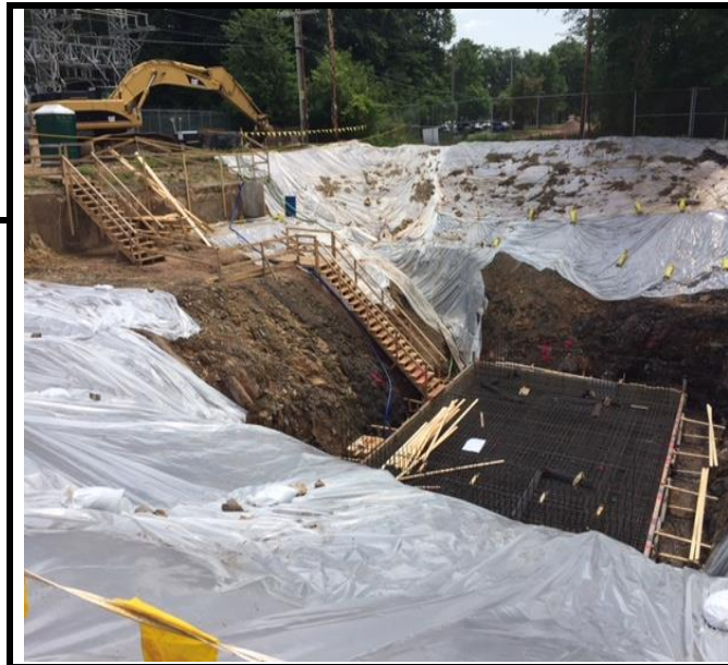
Footing and steel being installed at lift station
