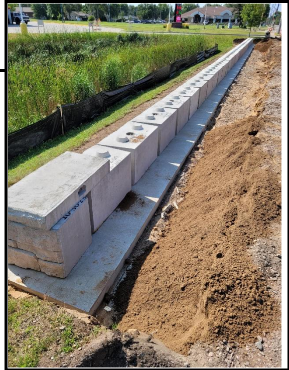
Retaining Wall on Lincoln Street
