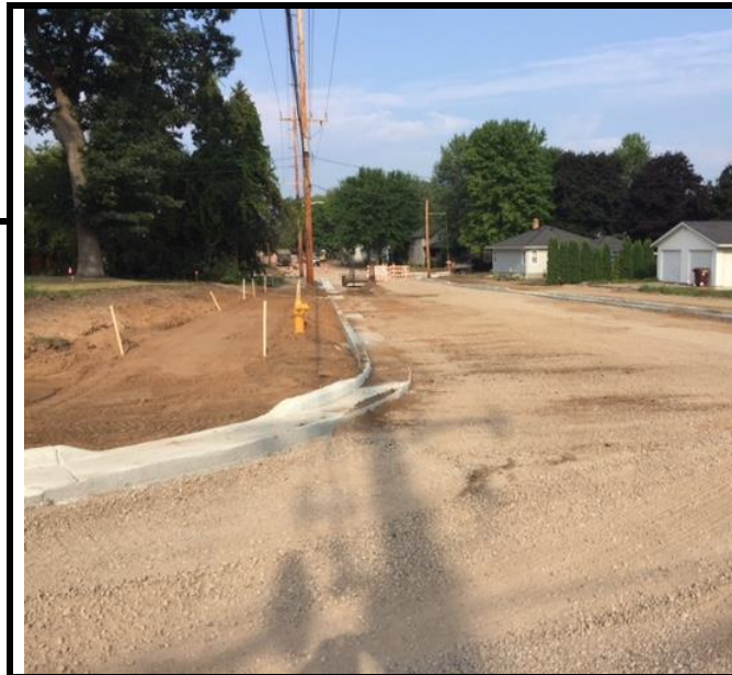
Curb complete on first section of High Street
