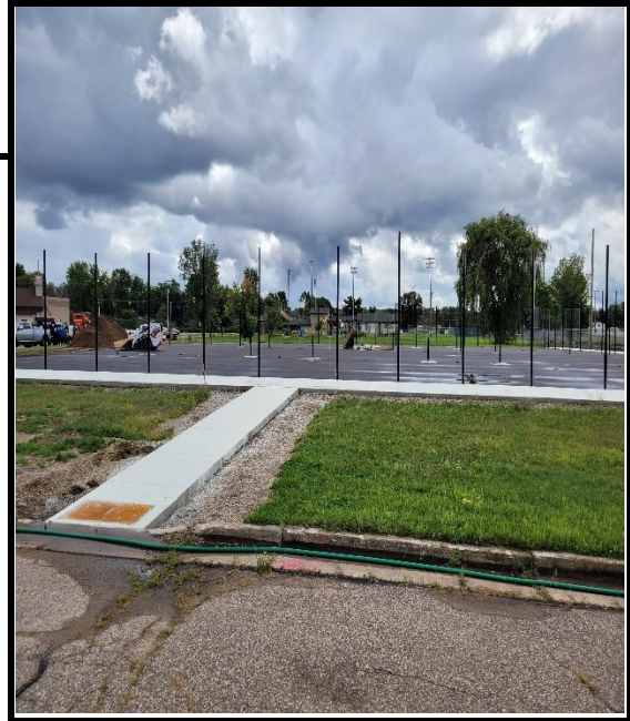
Pickleball Court Construction at Mead Field
