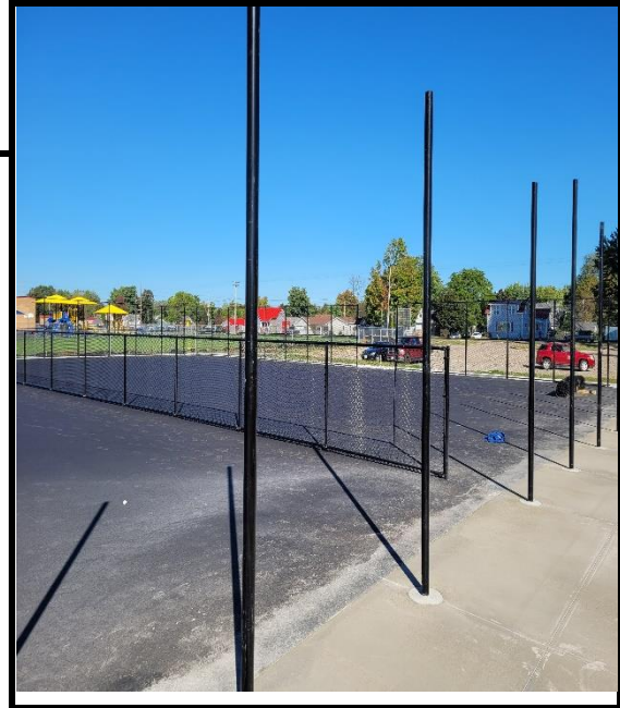
Pickleball Court Construction at Mead Field
