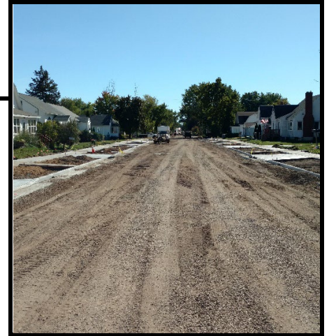
18 th Ave curb and gutter
