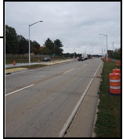
Expressway Concrete Repairs
