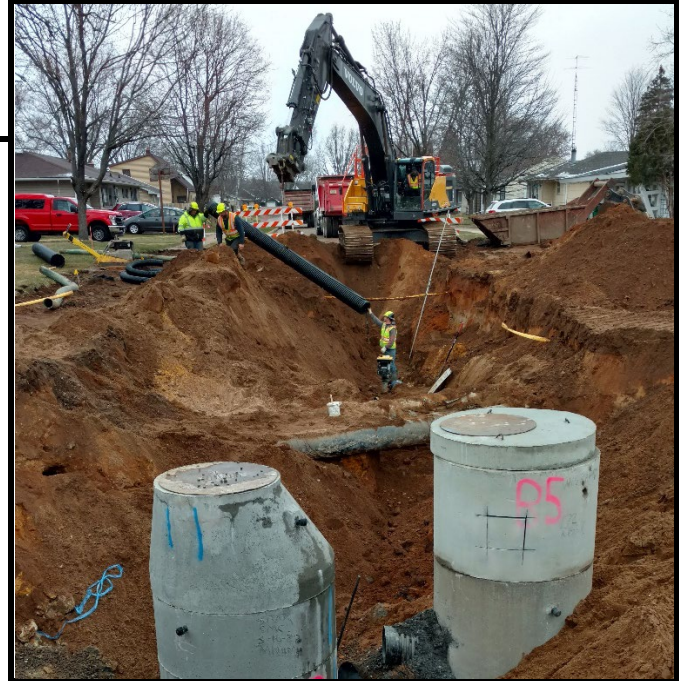
Cherry St – Storm Sewer Installation
