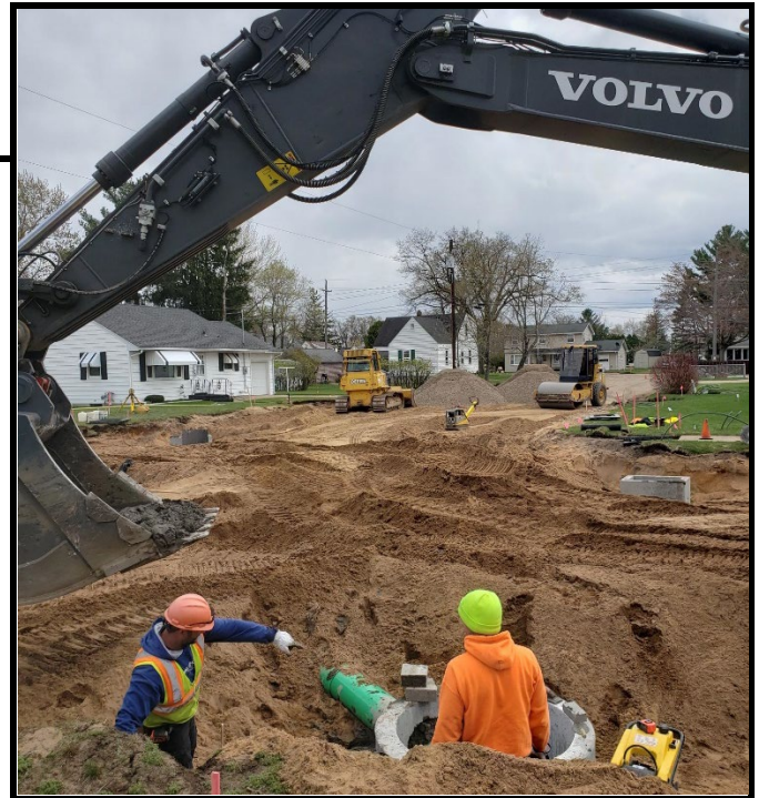
15 th St N Storm Sewer at Irving
