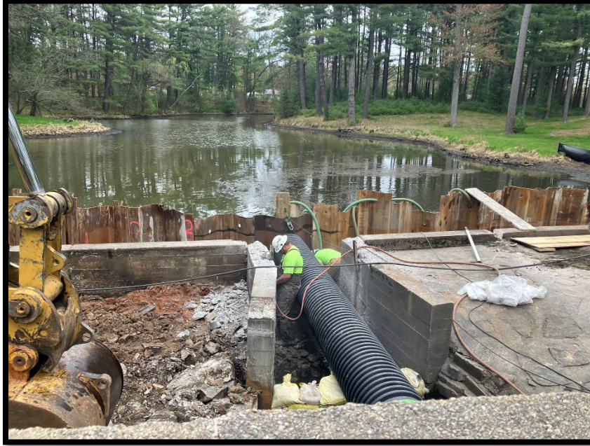
One Mile Creek Dam Repair
