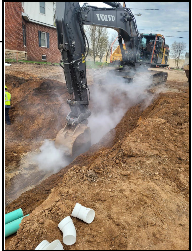
Sewer Installation on Plover St – looking west
