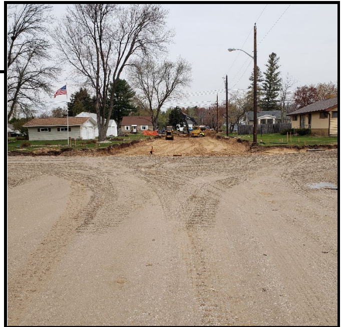
15 th St N Storm Sewer at Irving (looking north)
