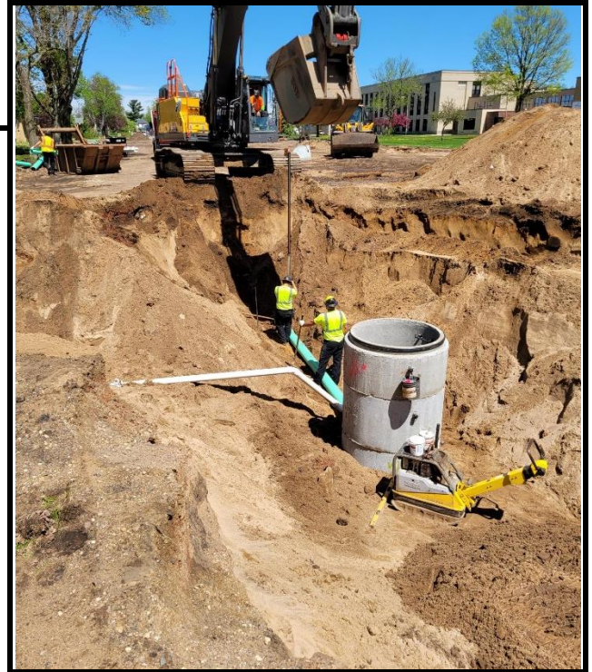
Lincoln Street north of Witter Street
