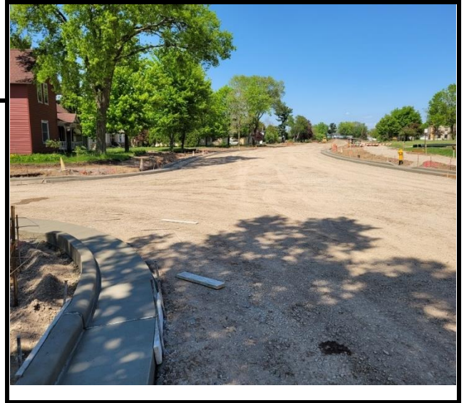
Lincoln Street Curb & Gutter
