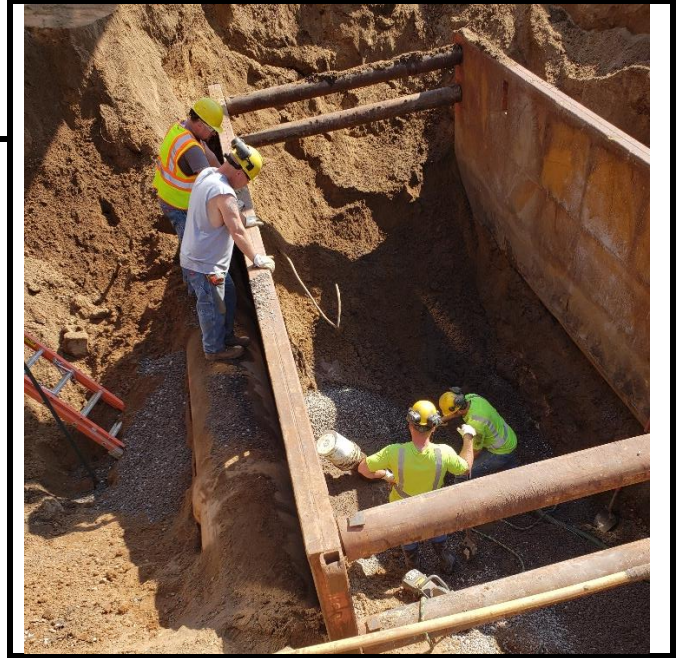
City Crews battle groundwater during sanitary lateral replacement
